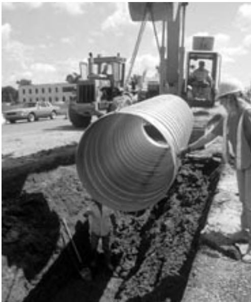
Reduced excavation because of ULTRA FLO's smaller outside diameter.
