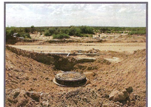
New Subdivision in Horizon City, Sanitary Manholes
