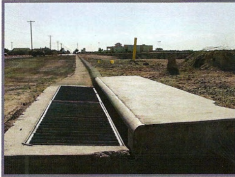
Target , Loop 375, Curb Inlets
