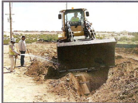
New Subdivision in Horizon City, Underground Sanitary Sewers
