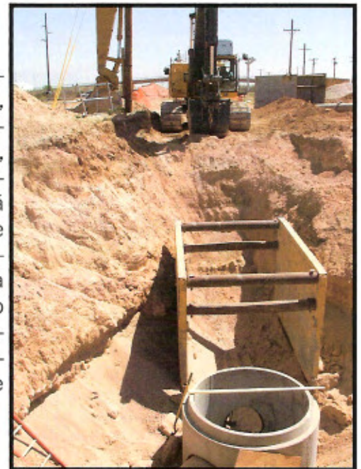
Manholes at Ft. Bliss being installed
