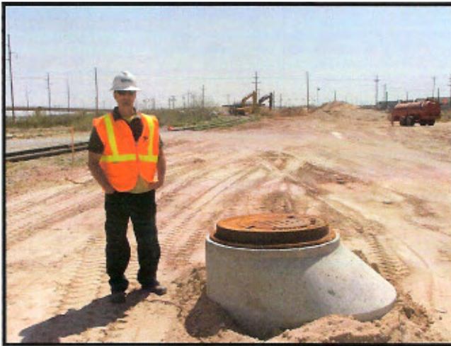
Keith Lemaster, Project Engineer of Garney Construction, at Ft. Bliss site
