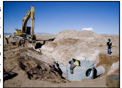
Installing Underground Manholes at Spur 601.
