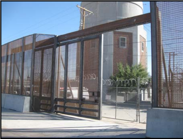
Concrete unit installed at Kiewit border fence site.
