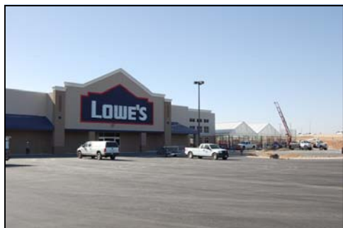
Lowes site off Zaragosa in El Paso
