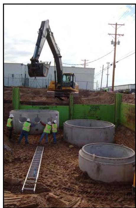
12 ft. ID Manhole installed at lift station.
