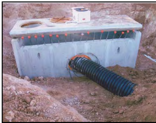
Precast Concrete Storm Sewer Inlet
