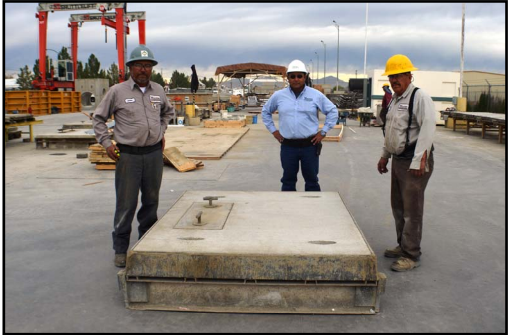
Ruben Rodriguez, Jorge Rodriguez, and Jose Carrillo clean an electrical transformer
