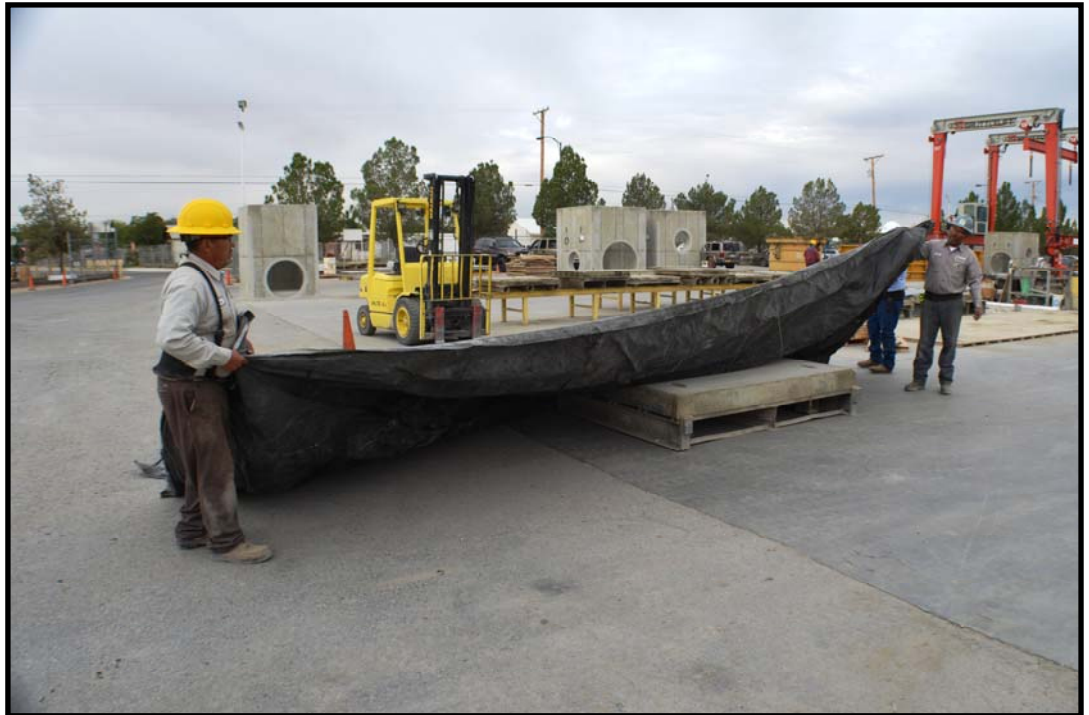
Product is covered to retain moisture while curing.
