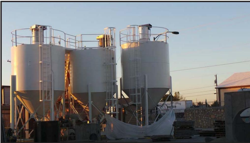
**A third silo used to store Type V cement was recently installed.**
