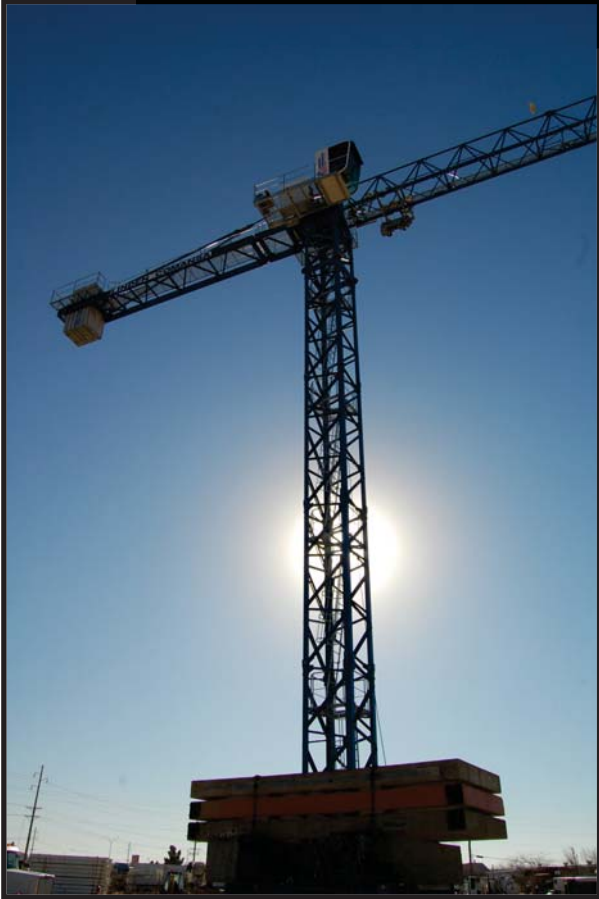
New Linden Comansa at Alliance yard.
