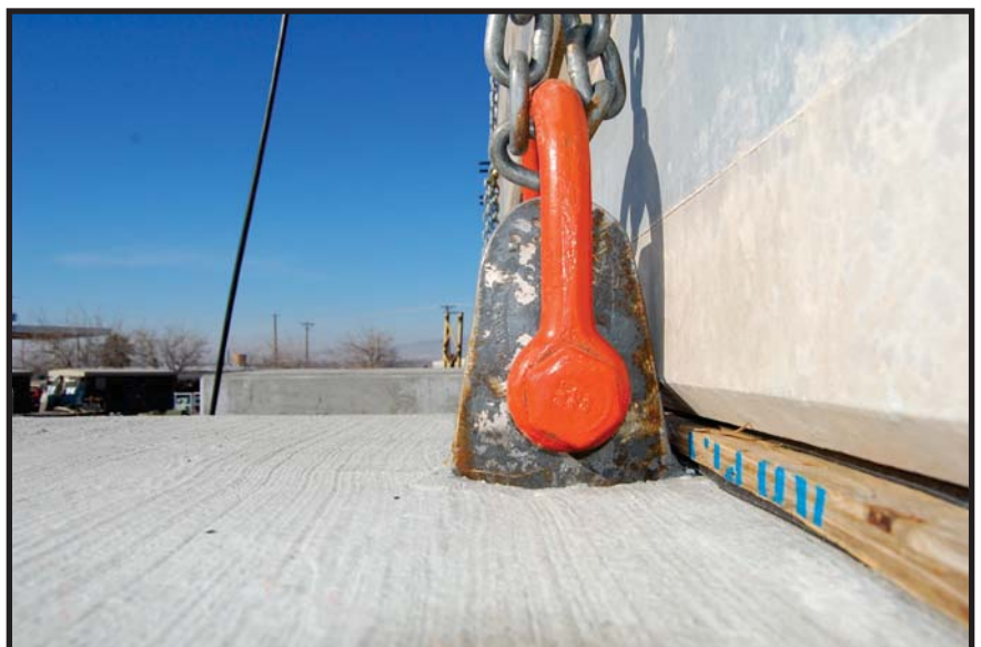
Concrete beam provided by Western Precast.
