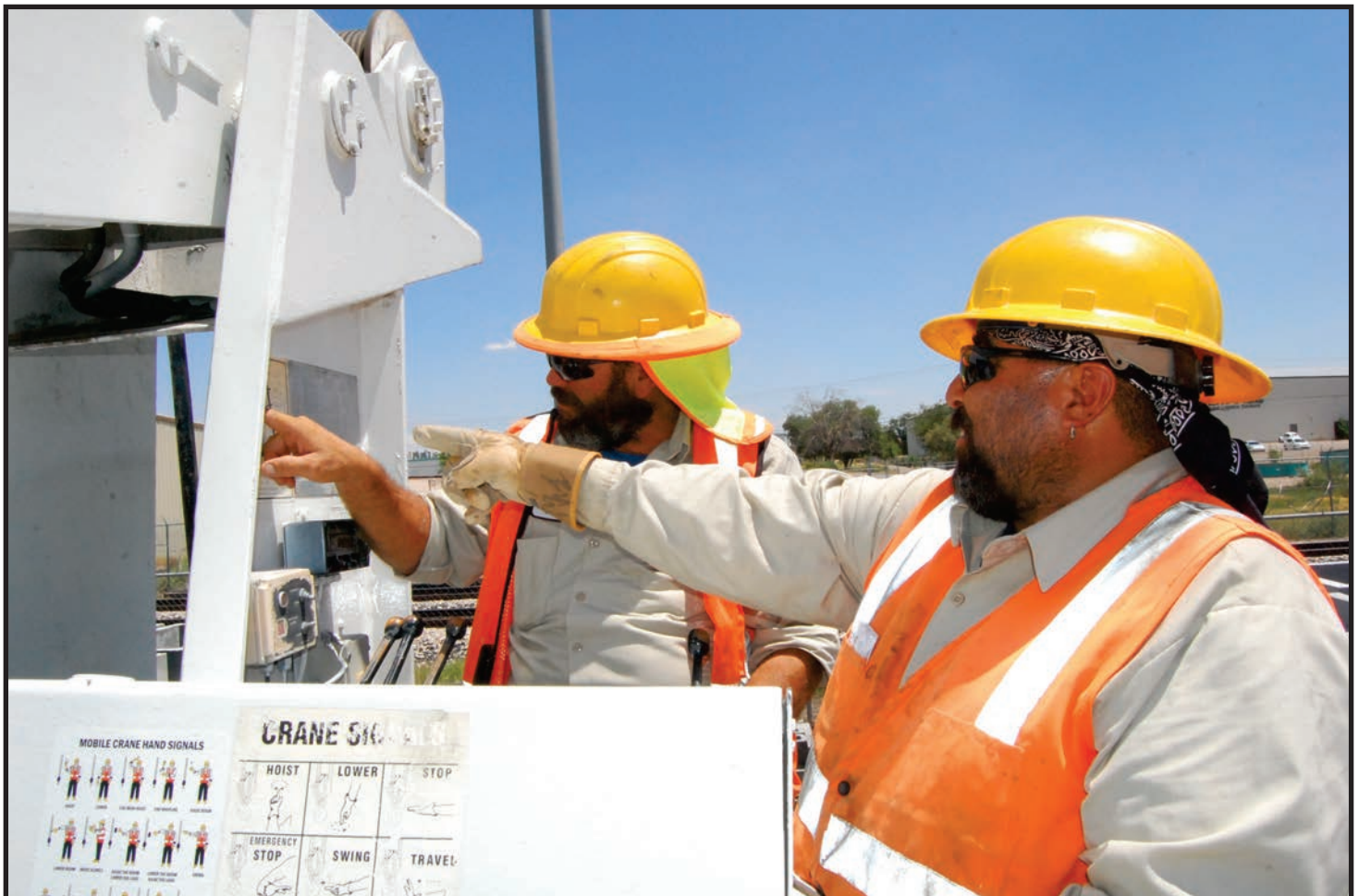
Jose Gomez and Victor Trujillo look over a crane load chart before operating the crane.
