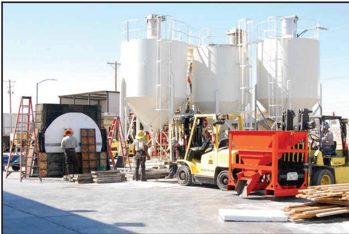
Western Precast Concrete plant operations located at 9101 Roseway.
