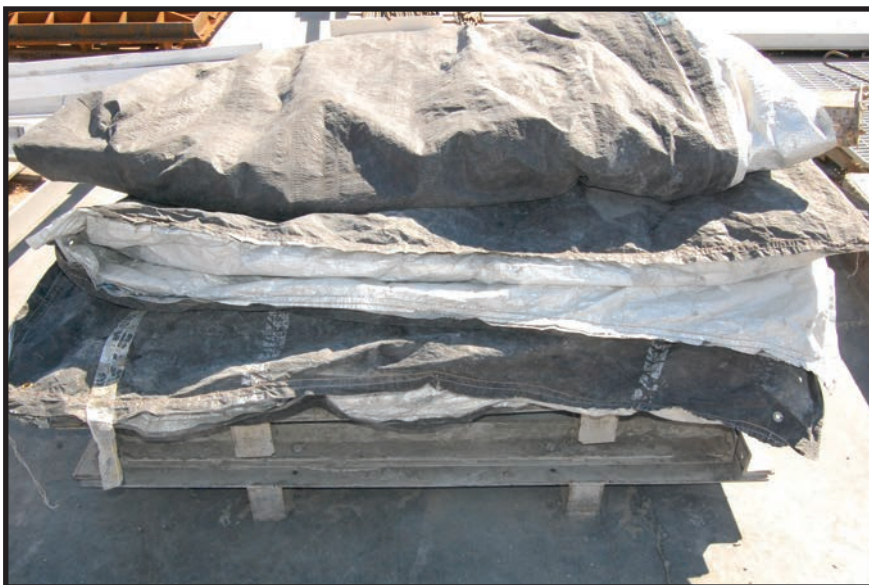
6 Curing blankets help to achieve strength in concrete.
