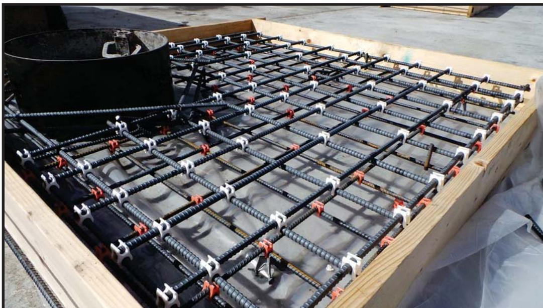
Properly placed rebar in form per specifications.
