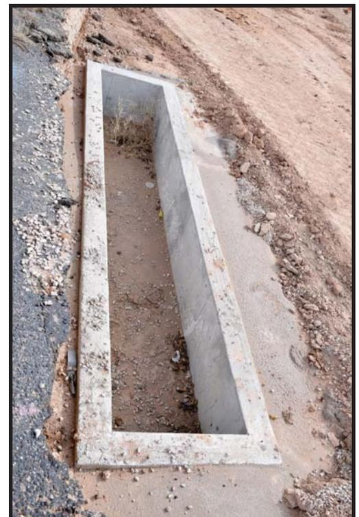
NMDOT type III B inlet installed at job site.
