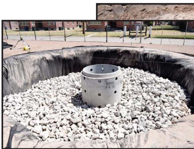
**French Drain type manhole used to collect and slowly disperse rain water collection from the general area.**
